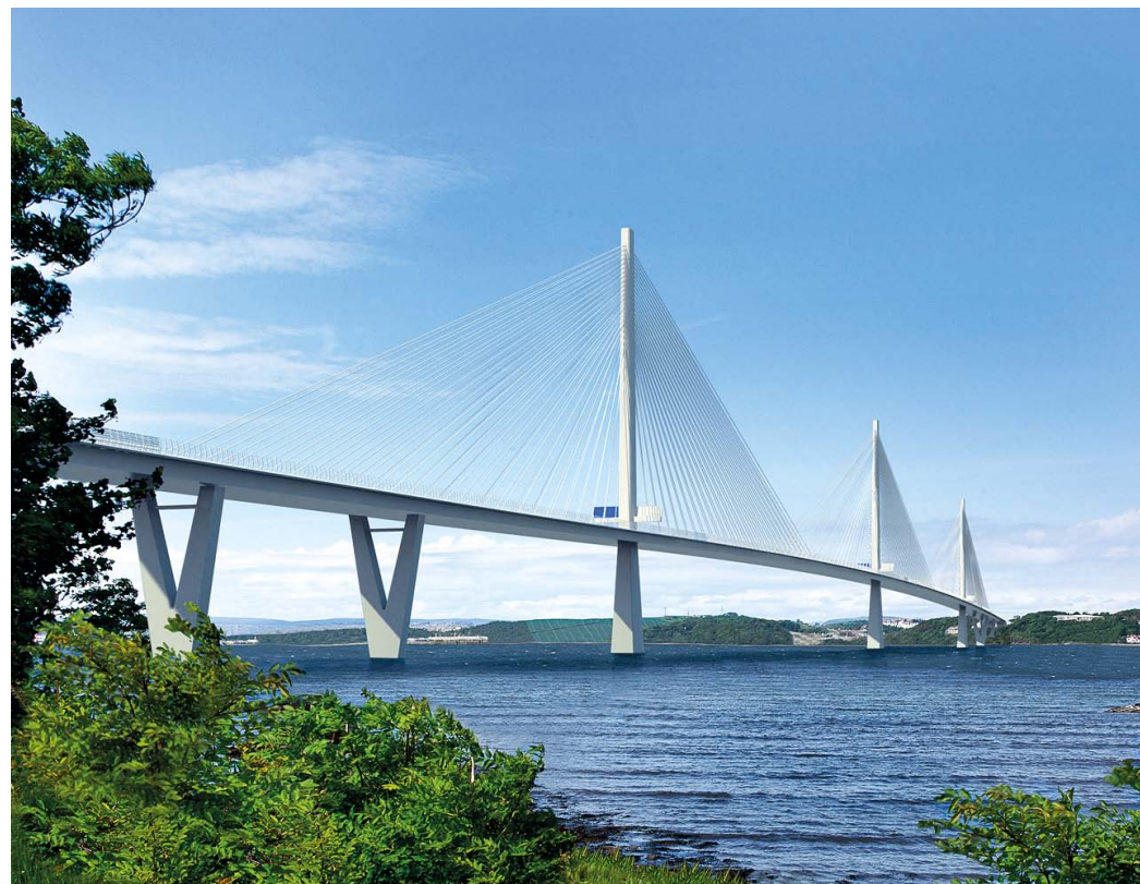
Forth Crossing Bridge
