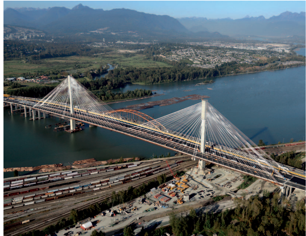
Port Mann Bridge, Vancouver
