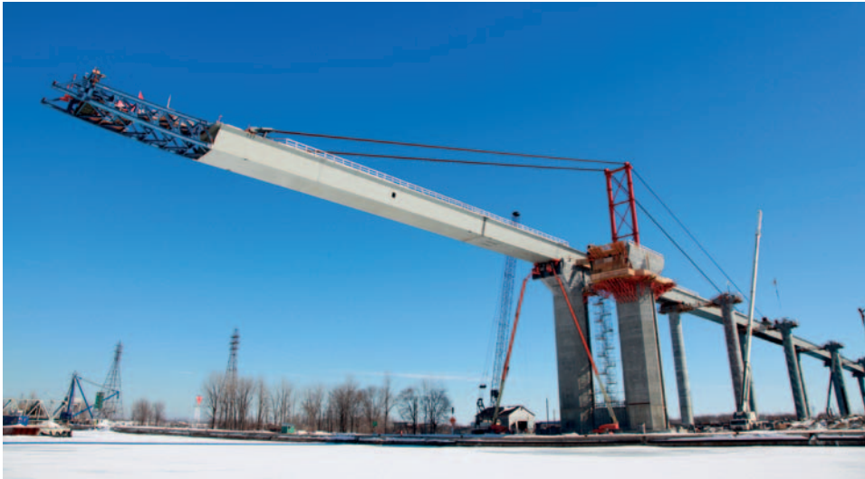
Canal bridge, NA30, Montreal Patrick Hally ©
