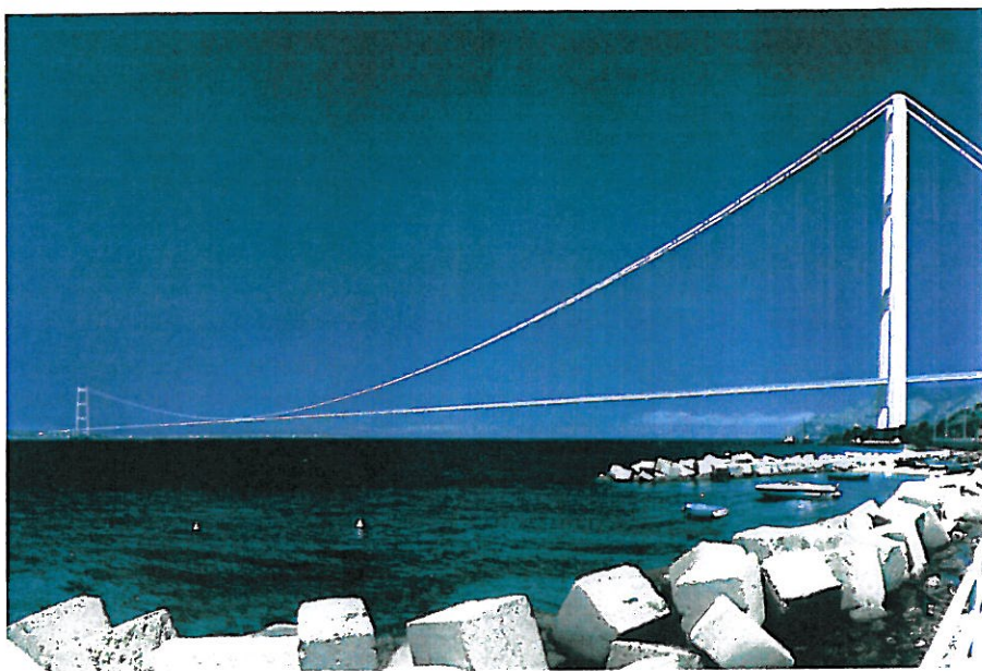
Strait of Messina Bridge (By permission of Stretto di Messina, Italy)
