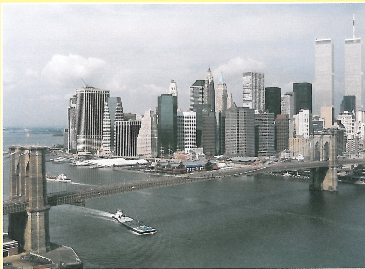
Brooklyn Bridge, Foto Bojidar S Yanev
